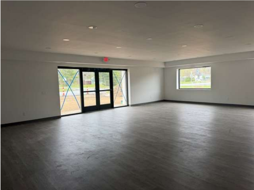
Suite 3 East Suite Front Section Looking North
